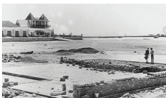
The foundation of the house (1966)
